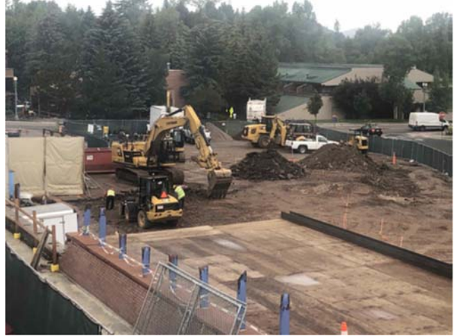
Asphalt demo in preparation for building excavation
