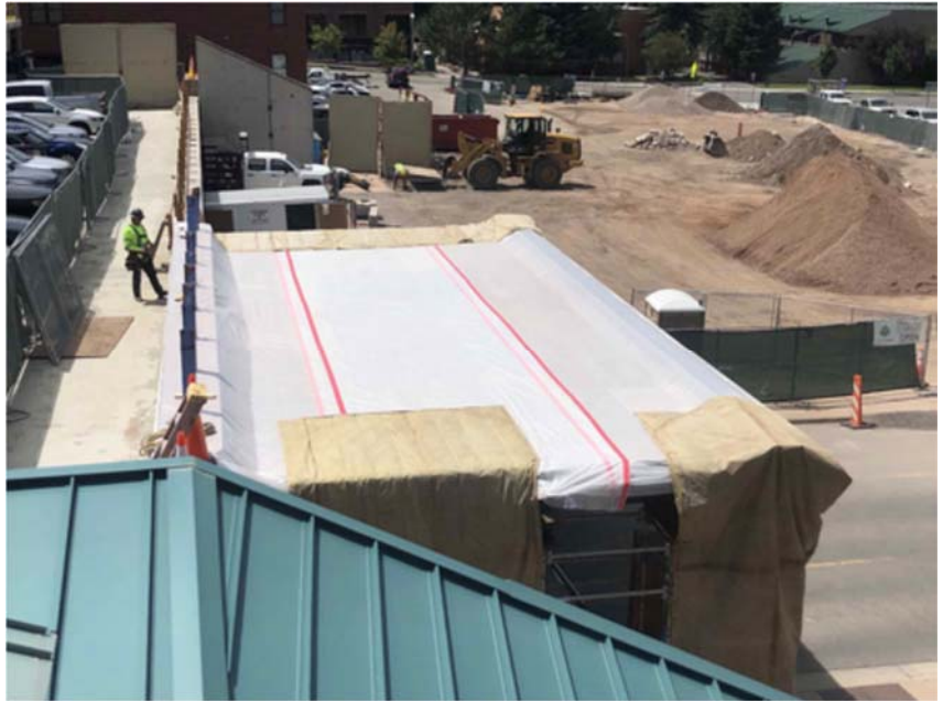
Plastic & sound blankets at garage entrance
