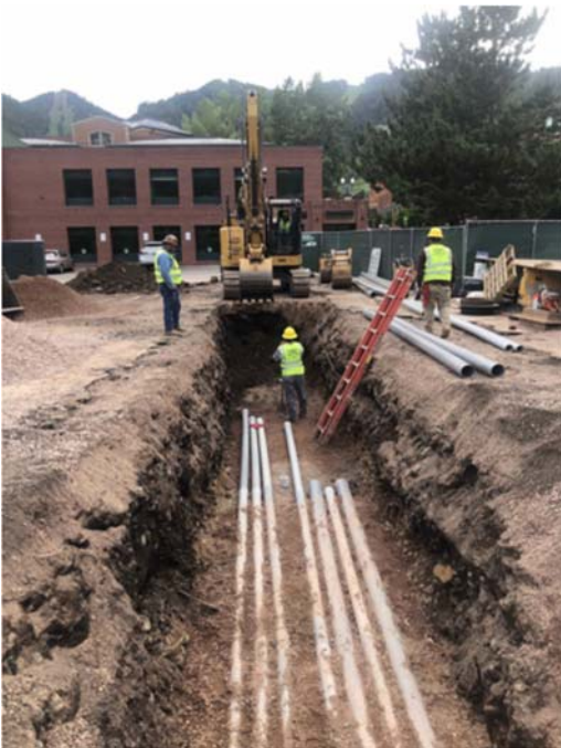
Conduits from the right of way onto the construction site
