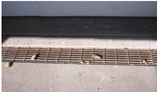
Figure 4.8 Trench Drain (Slotted Inlet) in City of Aspen
