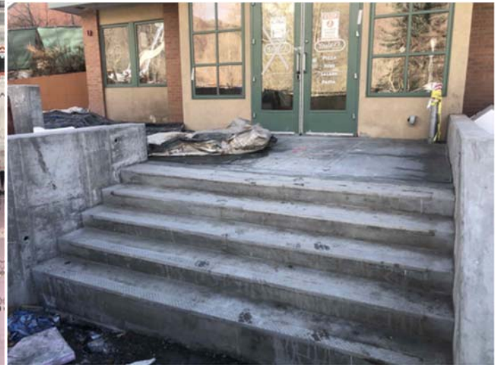
Taster's Patio stairs and slab placed
