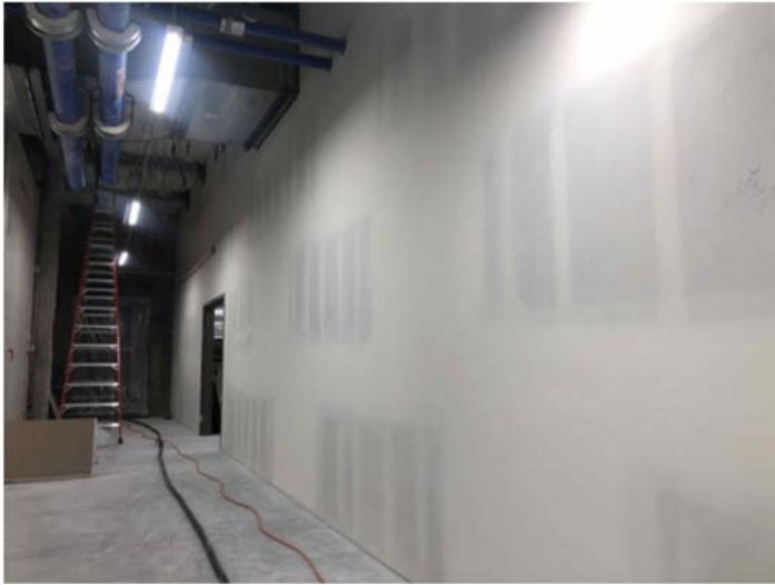
Basement tape and finish in progress
