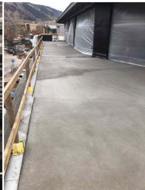
Phase 1 Plaza Topping Slab Complete
