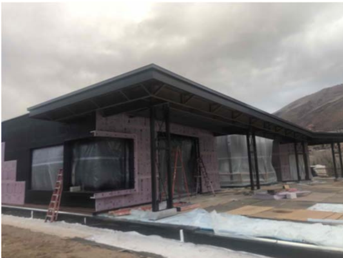
Upper level canopy and columns painted
