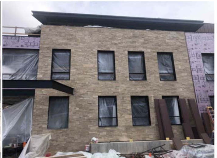
Stone veneer on west elevation complete
