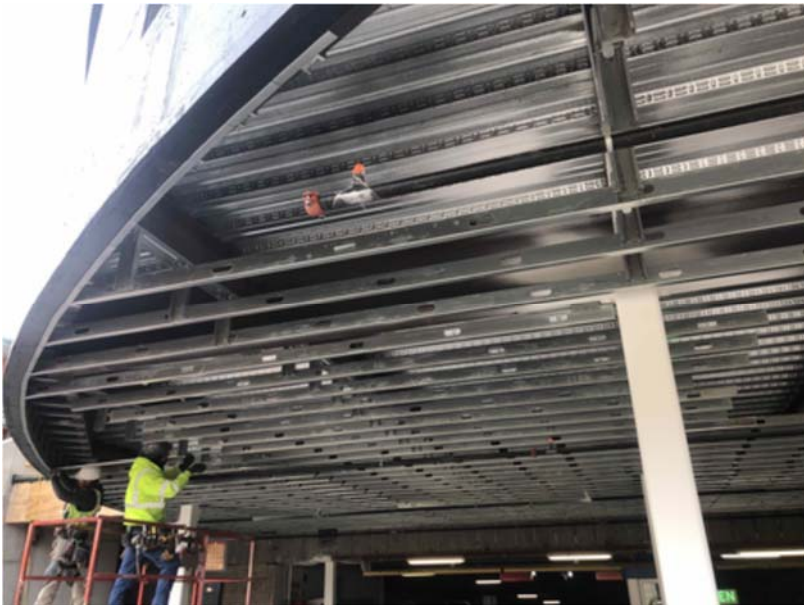
Garage entry soffit framing in progress
