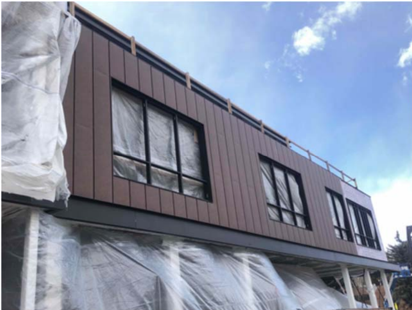
Storefront window frames – north elevation
