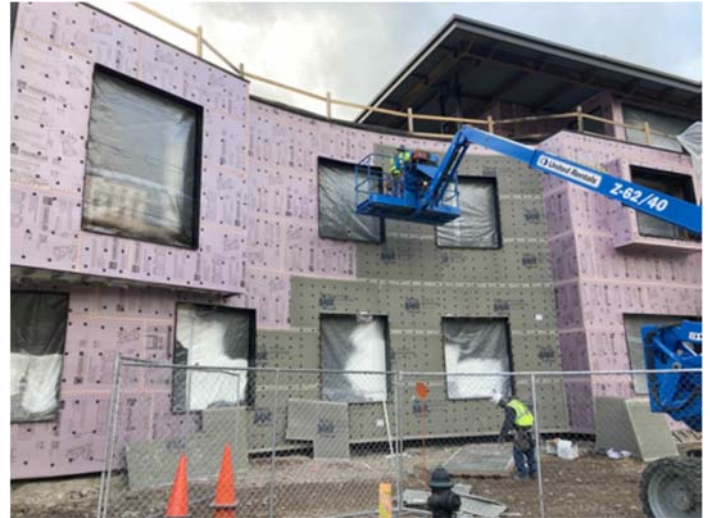
North elevation cement board progress
