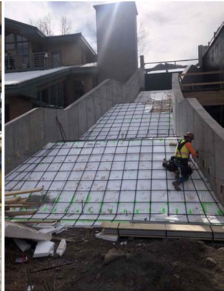
Grande Stair Geo-Foam complete
