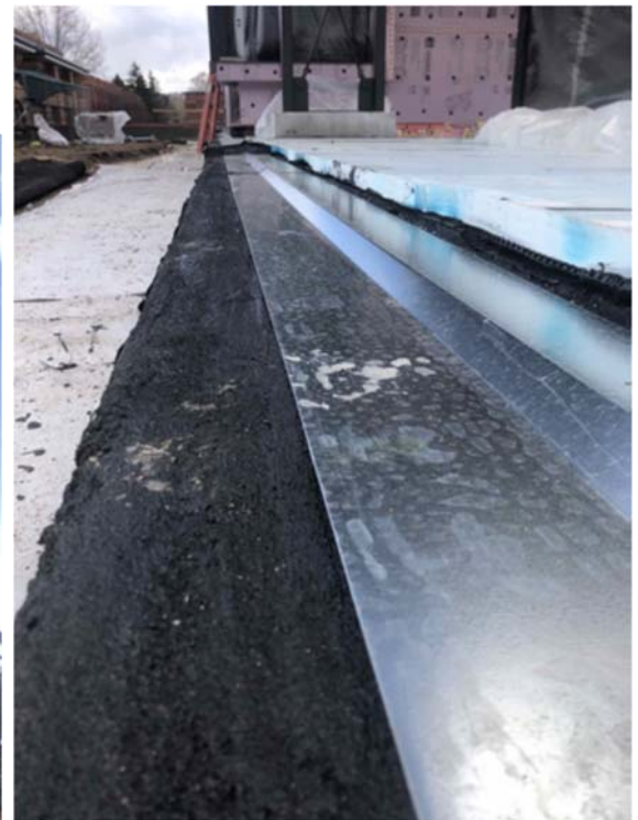
P6 waterproofing expansion joint complete
