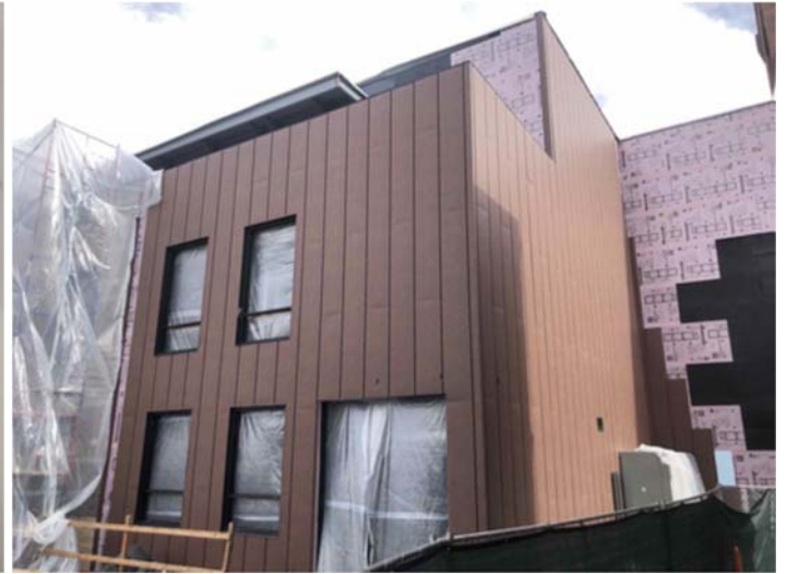
Metal Panel Progress
