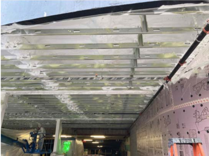
Garage entry soffit spray insulation complete
