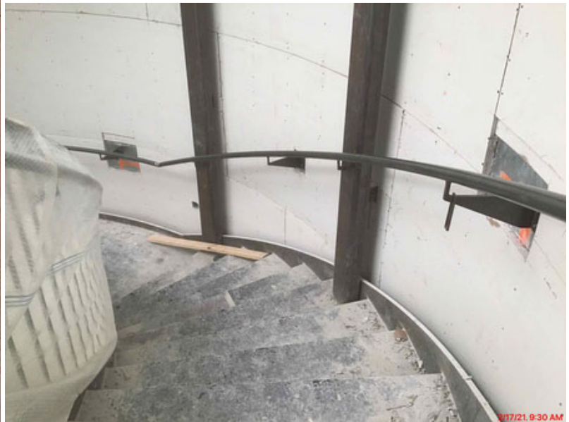
Install of radius stair railing complete
