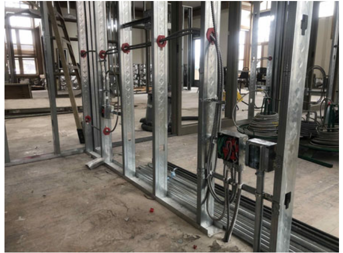
RGB Rough-in – in progress
