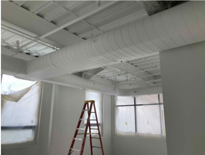
Overhead dryfall paint in progress
