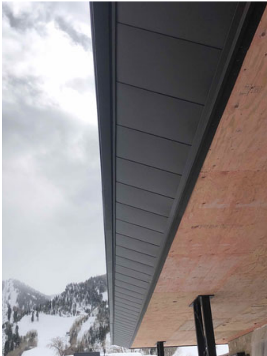
Upper-level canopy fascia metal in progress
