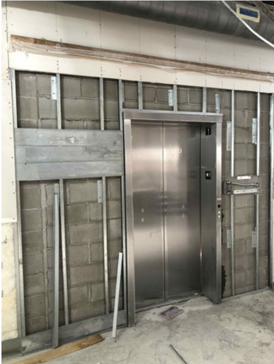
Elevator install complete – CMU infill around elevator Jambs complete
